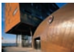
Centro svago urbano UEC, Almere, NL Will Alsop Architects, Londra Ridder Dak- en Wandsystemen BV, Hoorn TECU® Brass
