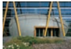
Centro amministrativo WeberHaus, Rheinau/Linxs, D Dipl.-Ing. Günter Hermann, Stoccarda Wittenauer GmbH, Sasbach TECU® Zinn
