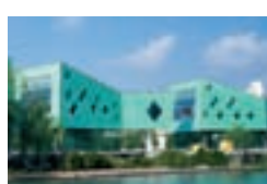
Yefei's Creative Street, Shanghai, VRC Will Alsop Architects, Londra, GB; U/Jiang Architects & Engineers, Shanghai Hanchang Industrial Development Co., Shanghai TECU® Patina, TECU® Oxid, TECU® Bronze
