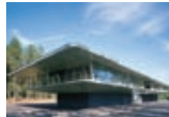
Centro operativo controllo traffico stradale VCNON, Wolfheze, NL De Architecten Cie, Amsterdam Verkoelen Dakbedekkingen BV, Beegden TECU® Zinn
